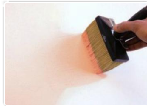
Step 4 - First coat by "pull and blend"
