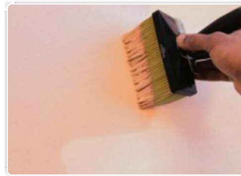
Step 5 - Second coat by "pull and blend"
