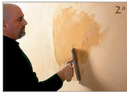
Step 4 - Second Coat, freely distribute the product with the trowel.
