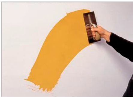
Step 3 - First Coat, freely distribute the product with the trowel.
