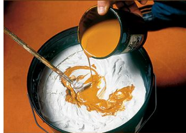
Step 2 - Prepare the shade with our paints indicated in the sample collection and mix with the beater; allow to rest for 24 hours.
