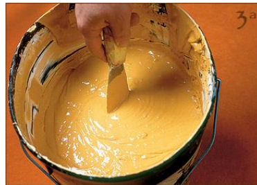
Step 5 - Third Coat, an important trick to achieve an easy polish is to mix Spatula Stuhhi well to make it more liquid.
