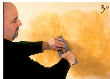
Step 8 - ... 30 seconds later we polish using a very clean spatula, in this way. We go on to the next square meter, overlapping the first to eliminate any sign of seams.
