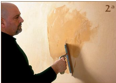
Step 4 - Second Coat, the surface is perfectly dry and absorbent giving a completely smooth surface, the ideal requisite for an excellent THIRD COAT.
