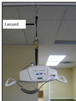
Figure 10A - Photo of lift hook connected to a P-600 lanyard first and then to the eyelet of the trolley.
