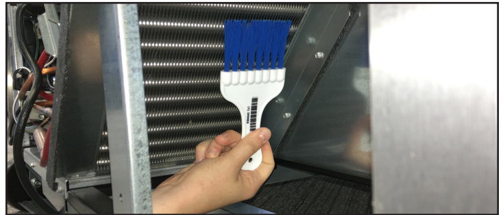
Fig. 3. Never brush across the coil fins.
