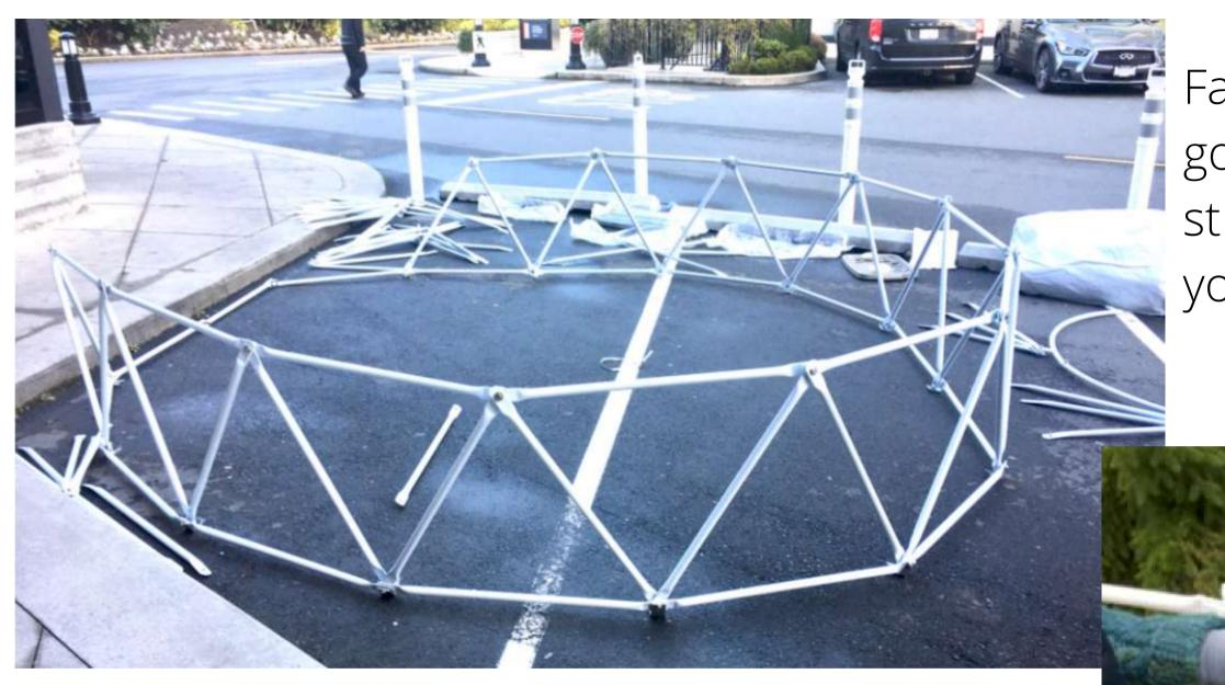
Fasten the first layer together- it is good to have 3 people to help hold the struts. Leave the nuts loose for now, as you will need to attach more struts still.
