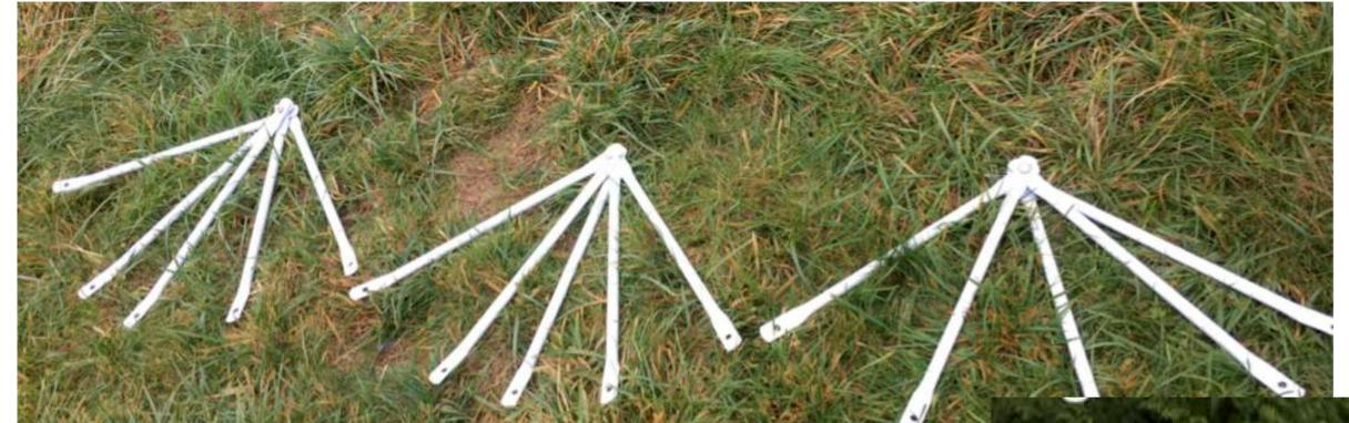
you can pre-assmble the 5-pointed stars on the ground loosely with a bolt to make it easier. Then attach them to the frame, letting the extra struts hang for now.
