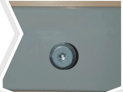
Insert nut inserted into the inside of the mattress side channel
