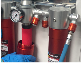
Unscrew lower section
