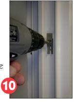
Using screws provided in Poly Bag #1, attach the hanger to the frame, keeping the hanger centered on frame (see Picture #10).
