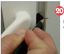
Partially close your sliding door so that you can mark the location of the top edge of Lock Catch inside your pet door frame. (see Picture #20)
