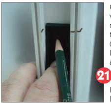
Open door, relocate Lock Catch to line up with pencil and mark holes (see Picture #21). Install Lock Catch using 1/4" self-tapping screws provided in Poly Bag #2. (see Picture #22) Use Spacer if needed. Lock Catch has slotted holes for adjustment if necessary.
