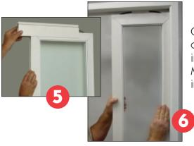
Carefully remove "H" Top Section from top of door. (see Picture #5) Place your pet door in position as shown. (see Picture #6). Make sure that the bottom Hanger on door is interlocked with Hanger on frame. (Picture #7)
