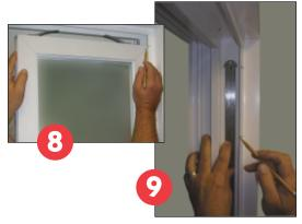
With pet door in place, mark a pencil line to correspond with top of door on edge of frame. (see Picture #8)
