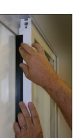
The Draft•Stopper™ attaches to the moving section of your sliding glass door. To install the Draft•Stopper™, measure the vertical distance, or height of exposed glass, between top and bottom frames of the sliding door. Cut Draft•Stopper™ to size with scissors using this length.
