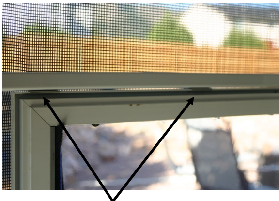
Interior and Exterior view of metal retainer clips attached to pet door and resting against spreader bar.
