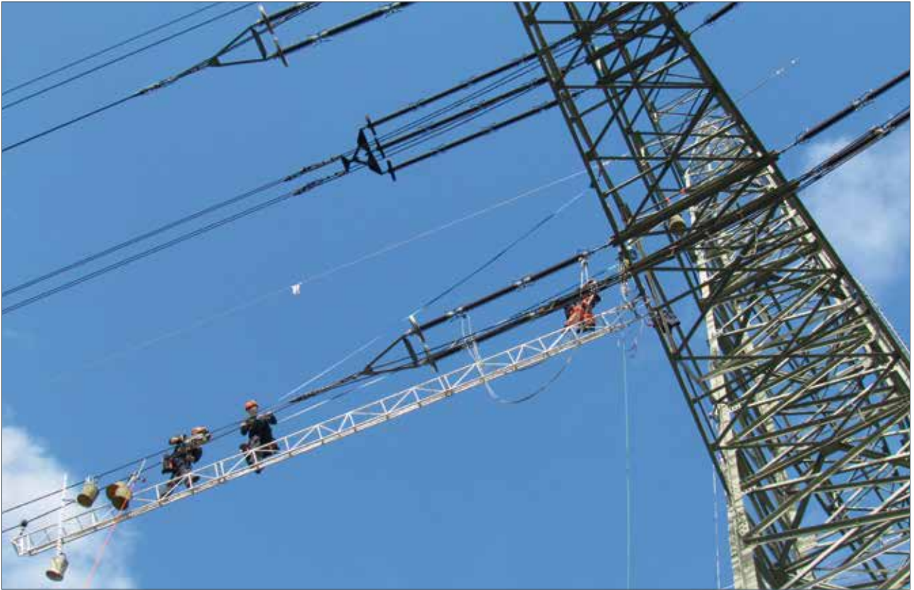
Overhead line construction
