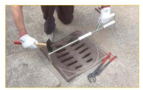
The beaks can also be used in the operations of scraping the frame of the lid.
