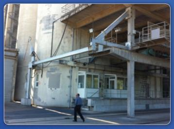
Raised COBRA PREMIUM. The custom-made support structure allows free passage of high vehicles under the rail.
