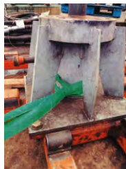
Figure 8. Typical Hitch on Valve
