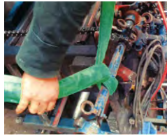
Figure 6. Choker Around Well Head
