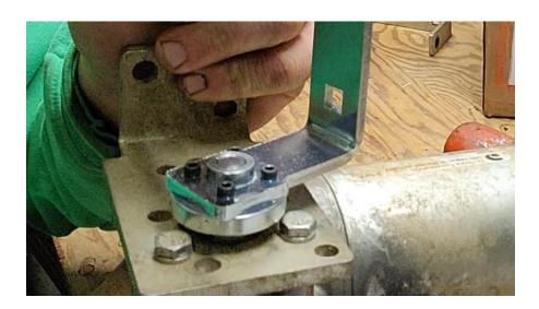
12.) Reattach other end of swing arm. Use included washers to fill the gap between the swing arm and the bearing. Install 3/8" bolt and secure with 3/8" Jam Lock Nut. Tighten using 9/16" Wrenches.
