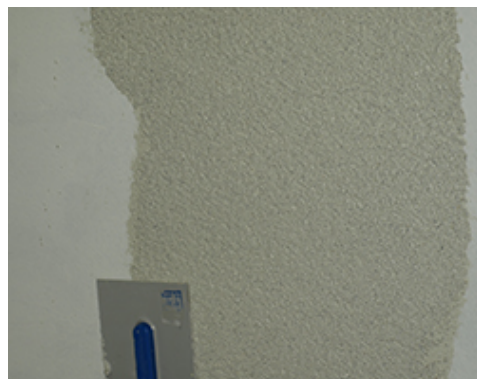
Trowelling: Trowel with a PVC
