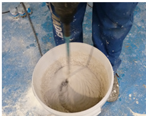
Mixing: Mix the plaster with 4,25 litres of clean water with a 25 kg bag of Planitop Mineral
