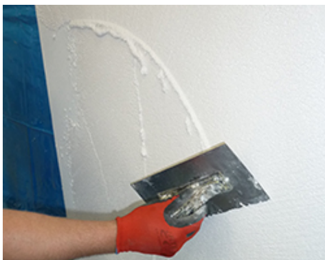
Application: Apply with a stainless steel trowel to the thickness of the grain
