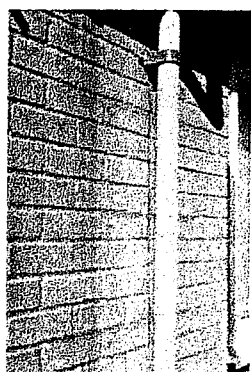
Movement Joint discreetly hidden behind downpipe
