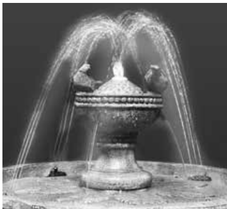
Correct position of the water spray nozzles.
