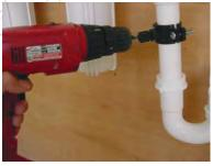
tubing to the fitting. Slip the nut over the tubing, and insert tubing into the drain saddle. This waste water is the life blood of the system. If the system cannot drain correctly it will not function for long. The system self flushing and the drain should never
