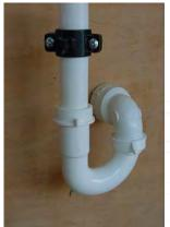
place 3-5" above the top of the bend in the P Trap. (See photo left) Again, just snug the drain saddle in place. Do not over tighten. Now drill a 1/8 to 1/4 inch hole thru the
