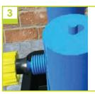
Remove collar Push 3/8" pipe through collar and attach to AQUAvalve5 nozzle
