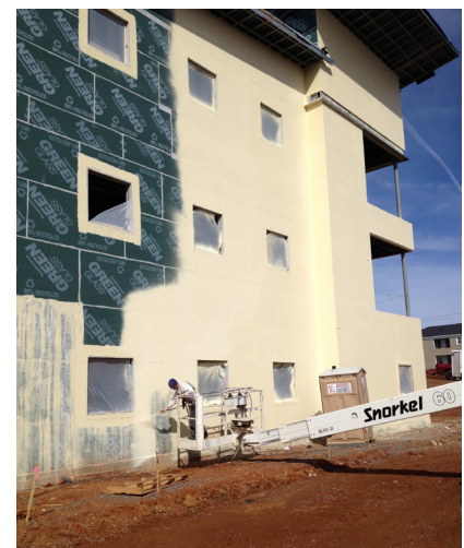
Application of Sikagard® 535
