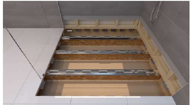
2. Attach Attach the new bracket system.
