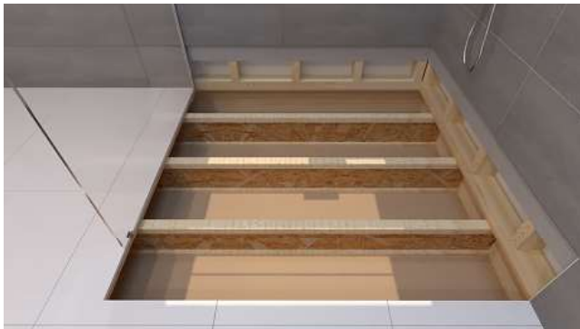
1. Expose Expose the joists.
