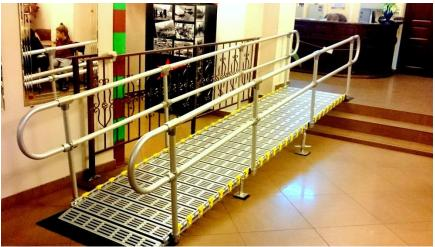
5 DEGREES SLOPE ANGLE (ADA-COMPLIANT 1:12 ratio): Height of location (inches) divided by 1
