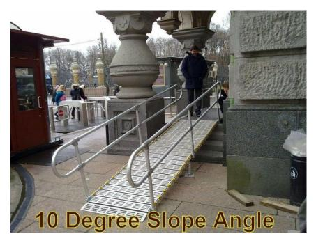
**10 DEGREES SLOPE ANGLE (1:6 ratio):** Height of location (inches) divided by a factor of 2
