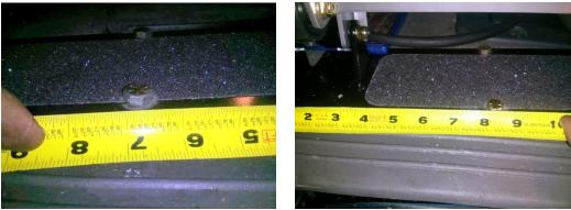
Position bolt 6 <sup>3</sup>/<sub>4</sub>" in from right side of bracket Position bolt 8 <sup>1</sup>/<sub>4</sub>" from left side of bracket
