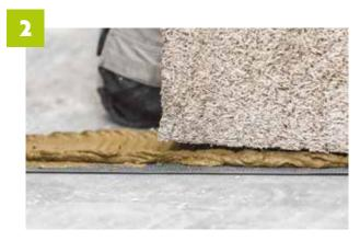
Apply a uniformly spread mortar bed 1 to 2 cm thick.
