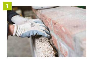
Manually fill in the space between the existing wall and the blocks gradually.
