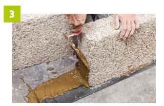
Glue the vertical joint and apply the next block. Adjust with a mallet if necessary to obtain a 3 mm vertical slim joint.
