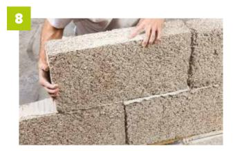
Place the block on the adhesive for masonry in 3 mm slim joints after taking care to glue the surfaces of the block (double gluing).
