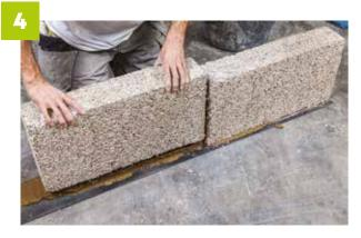
It is essential for this base course to be perfectly level. Check the perpendicularity and wait for the mortar to dry.
