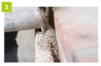
Use a light mixture of ProKalk lime and HempBag hemp according to the specification sheet, i.e. one bag of ProKalk for each HempBag.
