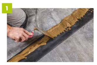
The IsoHemp blocks must be protected from capillary rise. Apply a sealing tape (of the DIBA type) going up 2 cm along the IsoHemp block.
