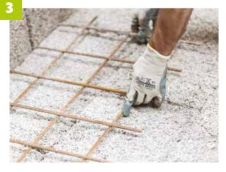
Lay a reinforced compression screed of min. 6 cm. This results in a surface ready to receive your finish of choice.
