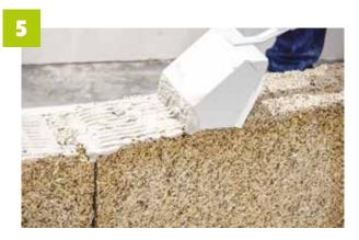
Apply the adhesive using a notched trowel over the entire horizontal surface of the already laid block to seal the joint.
