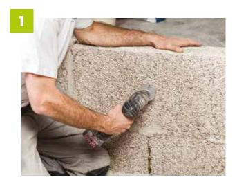
Drill the holes with a hole saw.
