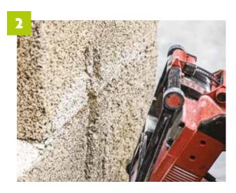
Create the grooves using a grooving machine.
