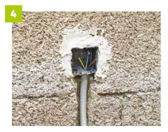
Fix the boxes and electrical cable ducts. Re-seal the channels and holes with a suitable sealant (natural plaster, etc.).
