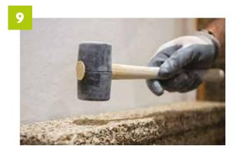
Adjust with a mallet and check the levels.
