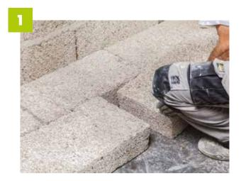
Check the tightness of the foundations before laying the block on stabilised soil or a concrete slab.
