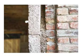
Do not leave any air gaps to avoid possible moisture problems at the interfaces of the different materials.
