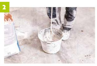
Prepare the Adhesive Mortar with 7 to 8 l of water per bag of 25 kg - usable for 1 hour.
