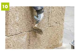
Remove excess adhesive using the trowel.
