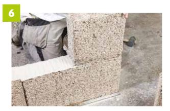
Lay the blocks in staggered joints (minimum 1/3 of the length of the block).
