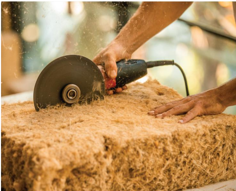
1 Insulation Cutting
