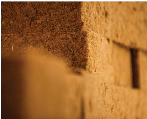
1 Prior to Installation
