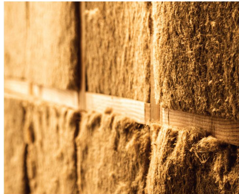
2 Installing Insulation Between studs
