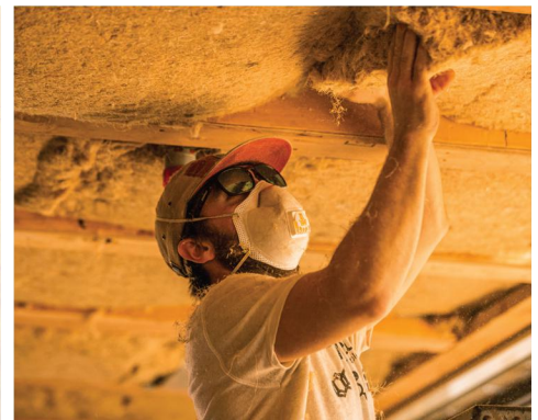
3 Possible Second Layer (Cross-Jointed)
