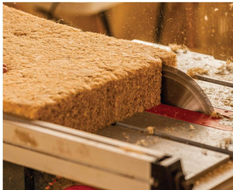
2 Cutting the Insulation
