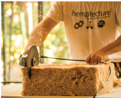
1 Prior to Installation
