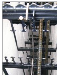
Vertical & Horizontal Clips in place close to corner
