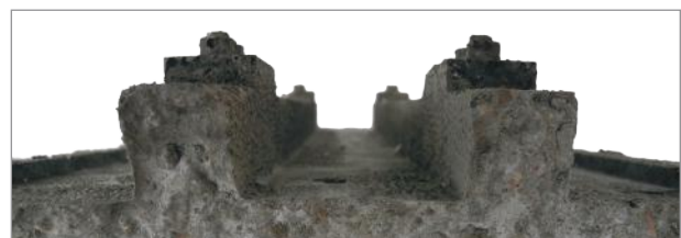
Photo above reveals consolidated concrete barriers created within the Fox Buck
