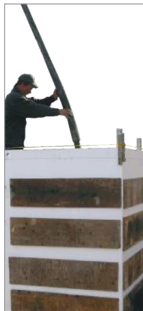
Some competitive ICF strap corners with lumber for strength during concrete placement.
