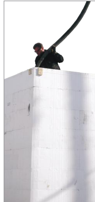
The Fox Blocks extended 90° corner block showing it's stand alone strength during concrete placement.
