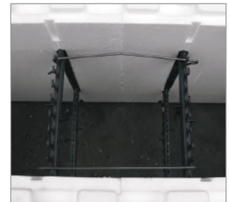
Horizontal Clips in Place
