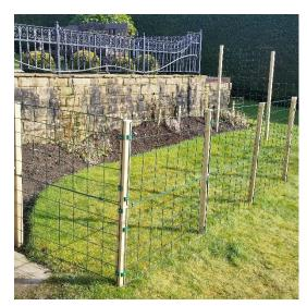
If the fence is going to be erected in a straight line and the end panel is to long simply bend the panel at right-angles to the exact length, do NOT cut the panel down.
