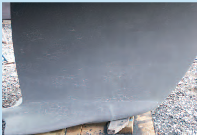
Antifouling paint cracking over the primer: This is caused by applying the antifouling paint to the primer before the primer has cured.
