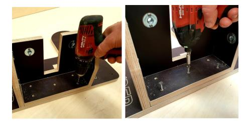
Next drill the two REAR holes directly behind the vertical plate. These may need to be at a slight angle as it can be difficult depending on the drill you have to make a vertical hole. Use the remaining two 4 x 30 screws. BEWARE of rounding the Screw Heads! CHECK all around the structure to make sure it has pulled flush with the base.
