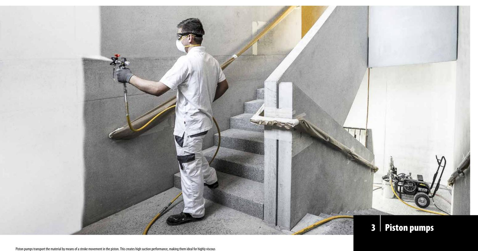
Piston pumps transport the material by means of a stroke movement in the piston. This creates high suction performance, making them ideal for highly viscous materials. Pneumatically driven piston pumps are explosion-proof and therefore suitable for use in workshops. Our hydraulic piston pumps offer even greater performance and can also be operated with petrol.
