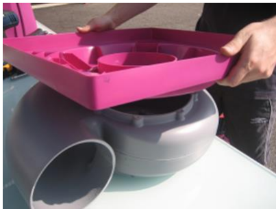
10. Place the roof curb cap on the housing.
