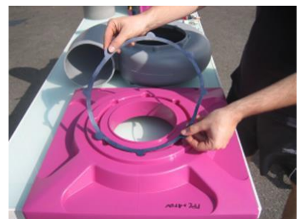
9. Place the roof curb cap O-ring seal.
