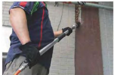
Corrosion removal for inaccessible area
