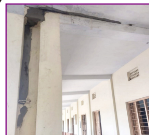
Repairs were completed on all the water leaks
