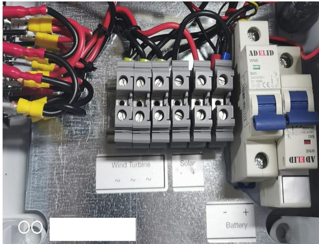
The controller has the following connections:
