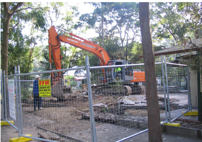
2.06.2005 the termite damaged building being demolished.
