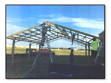
**10. Install fascia.** Trim purlin ends if necessary, at both ends of the gable so they are in line. Angle cut I x 6 treated fascia boards at the peak and eave, cutting to proper length. Nail fascia boards to the end of each purlin using 12-penny nails (provided by customer).
