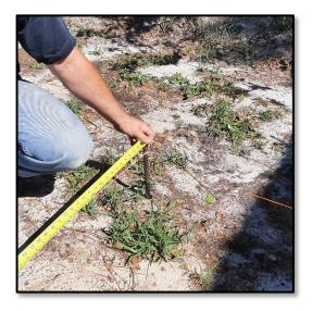
1. Lay out column placement. Mark the ground where your column will go, with stakes or paint. Most column spacing is 12', 10' or 8' so you will need two rows or marked column locations, with the appropriate spacing.
