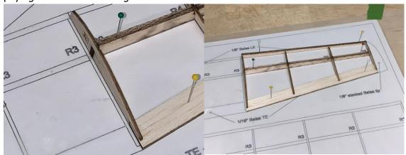
18. Remove the tip panel from the board and sand the R3 and R6 ends flush.
