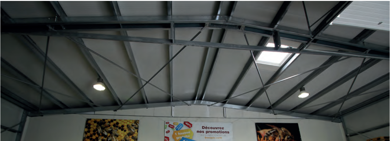
Jl Roof PIR as a kit-building in Seine-Maritime.
