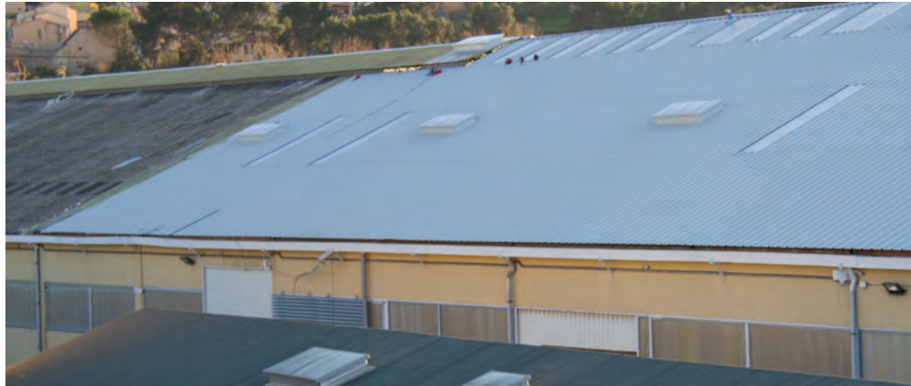
JI Roof PIR used in a renovation project.
