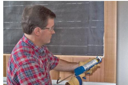
Proper Caulk Placement:
