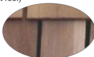
Exposed interlaid felt
