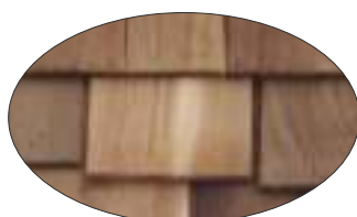
Uneven courses (on non-staggered butt roof)
