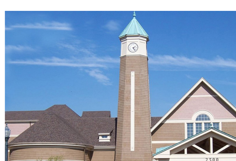
Project: The Glen Senior Living - Classic Residence by Hyatt Location: Chicago, IL Architect: Solomon Cordwell Buenz Co. - Chicago, IL Builder: JC Inc - Wheaton, IL Product: 7-1/8" Even Keyway Color: Rose Quartz & Taupe
