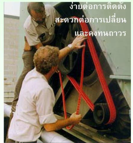
Cooling Tower Drive Installation
