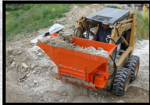
Step 2: Level Hog Crusher and start recycle process.
