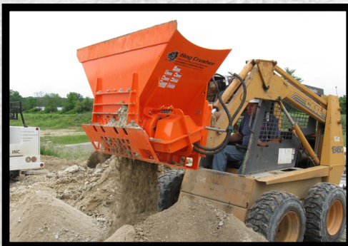
Step 3: Powerful Hog Crusher pulverizes debris in minutes.
