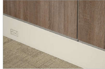
6" Vinyl Base accommodates horizontal modular power.
