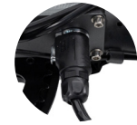
Battery connected to controller
