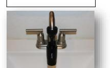
**4.** Attach flush bulb assembly to the sink faucet, slowly turn on water until a thin stream of water begins to flow. Flush for five minutes.
