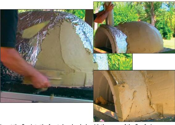
Insert the flue into the front chamber hole with the seam of the flue facing the back of the oven before beginning the rendering process. Use a spirit level to ensure the flue remains straight. For best results, use a steel float to apply the render mix.
