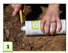
Cut the sealing cap off of the SPLAT Verb caulking tube.
